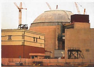
SUSPECT Russian-built Bushehr nuclear power reactor in southwestern Iran
